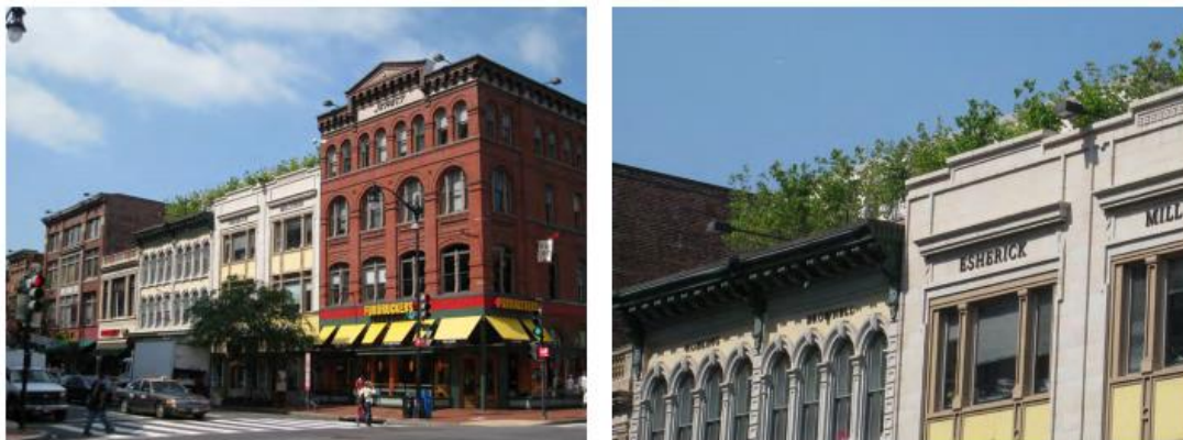
Figure 6 - Incompatible solution: the plantings were highly visible above the parapet wall (source: Petrella, 2009).
