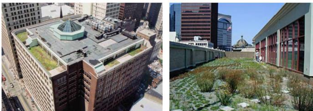
Figure 6 - Incompatible solution: the plantings were highly visible above the parapet wall (source: Petrella, 2009).
